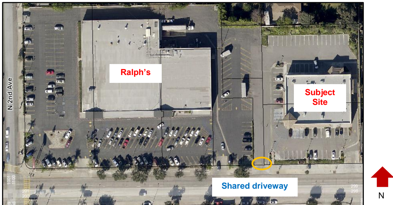
Figure No. 1: Ariel view of the subject site and the adjoining site to the west.
