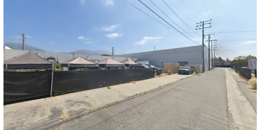
4 SITE PHOTO - VIEW FROM ALLEY
