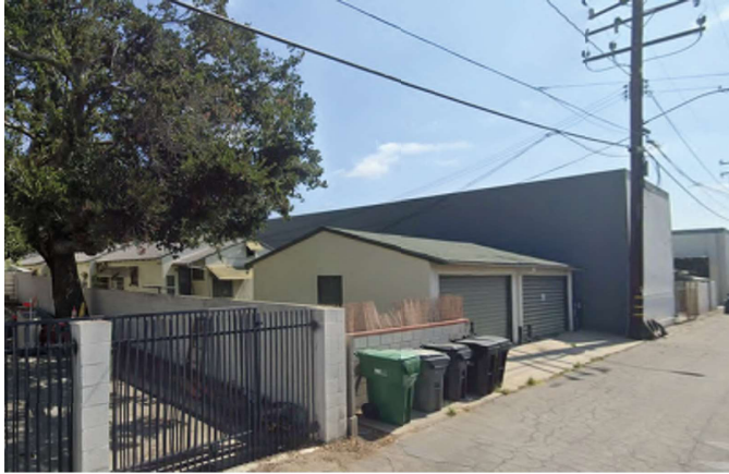
5 SITE PHOTO - VIEW FROM SOUTHWEST SIDE
