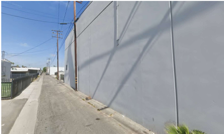
3 SITE PHOTO - VIEW FROM ALLEY
