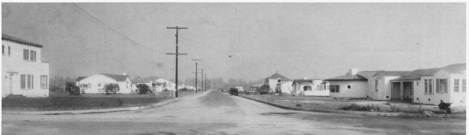
Looking east on Norman Ave. toward Santa Anita Ave., November 1936. This was part of the Baldwin Stocker Acres development and shows the houses near completion.
