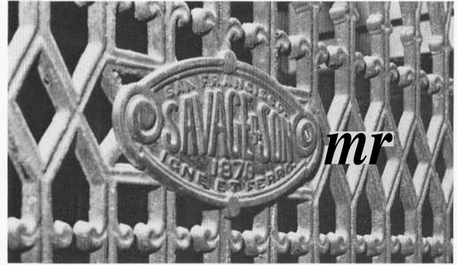
Baldwin Coach Barn ironwork. Manufactured in San Francisco in 1879, the ironwork in the elaborate Baldwin Barn complimented such additional interior detailing as redwood and cedar wall panelling and acorn-shaped stall finials.
