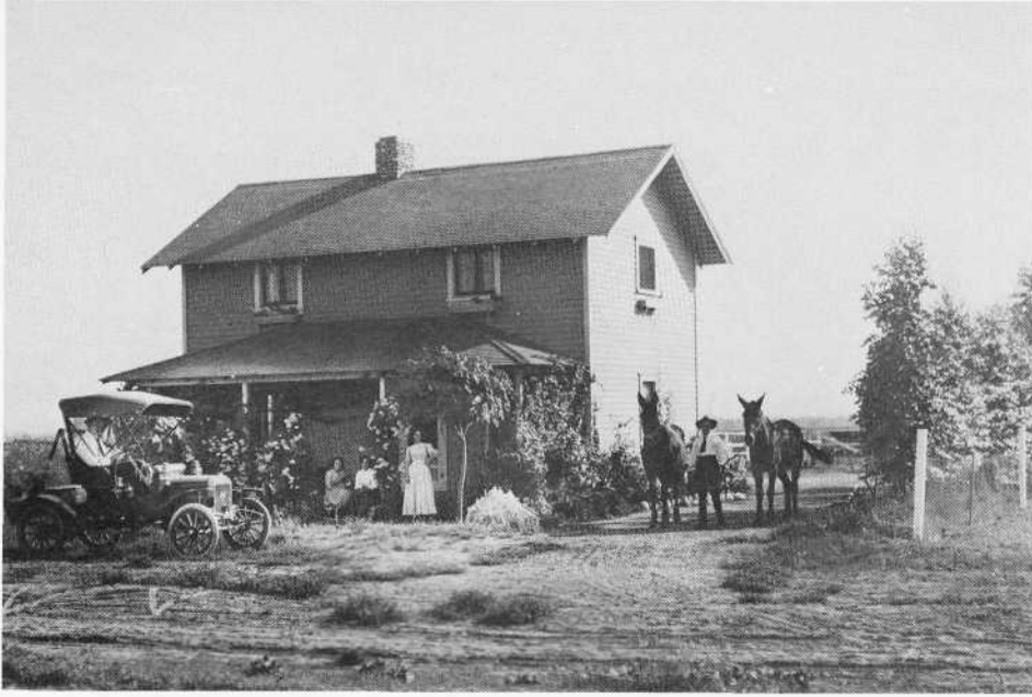
Home of William Millard on the corner of Sixth Ave. and Camino Real Ave., circa 1910. The building was destroyed by fire in 1970. — HELEN O. SCHRADER
