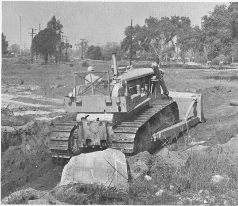
Bulldozer begins earth movement for the construction of the Foothill Freeway through Arcadia, 1967. — ARCADIA TRIBUNE
