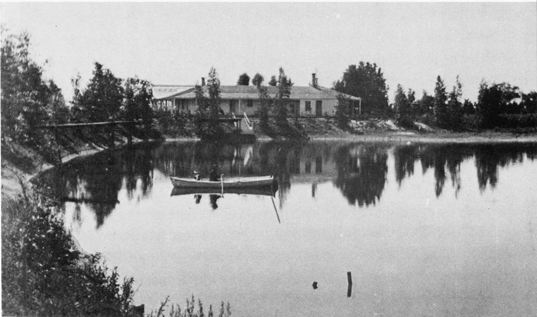
Lakeside view of the Baldwin Adobe and nearby greenhouse, circa 1878. The old three-room Hugo Reid Adobe (with Joseph Rowe's L-shaped addition) was renovated by Lucky Baldwin into a comfortable, up-to-date home. The lake served as a holding reservoir (note the pipes extending over the water) for Baldwin's irrigation projects in the early years. — THE HUNTINGTON LIBRARY — SAN MARINO
