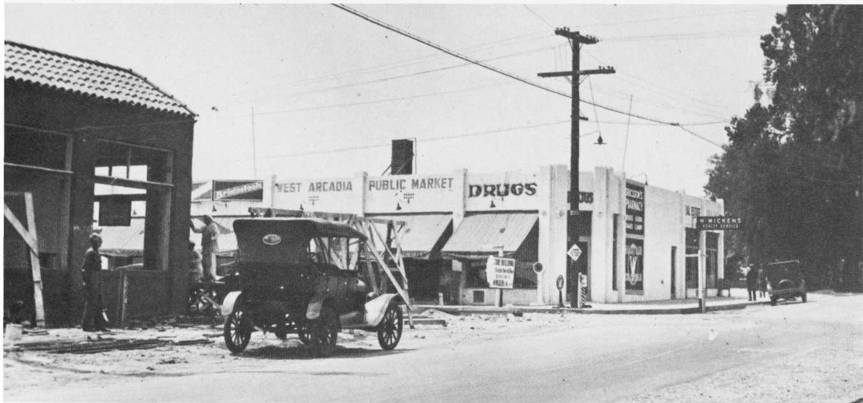
Looking west on Duarte Rd. into intersection of Duarte Rd. and Baldwin Ave., circa 1924. Ericsson's Drug Store appears where Hinshaw's Department Store stands today. The large building still under construction will house the Bank of Italy National Trust and Savings. Mr. McMicken's real estate office is on Duarte Rd. to the west.
