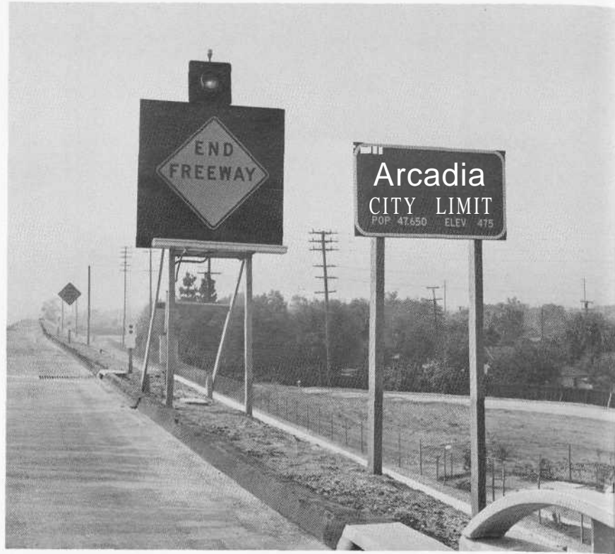
Foothill Freeway nearing completion. Eight lanes of concrete sweeping across the city have brought it irrevocably into the urban milieu of Southern California.
