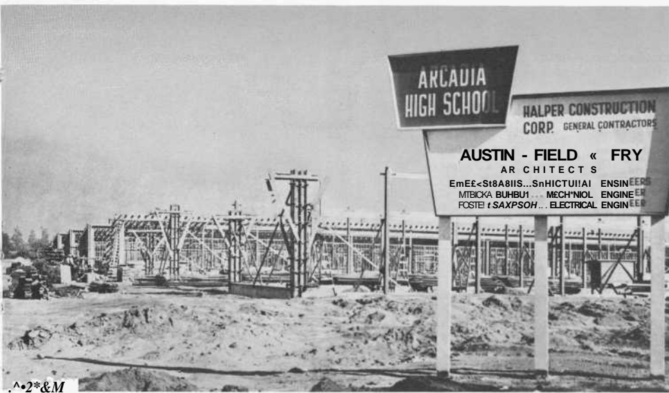
Arcadia's first high school under construction, late 1951. Classes opened in September 1952.
